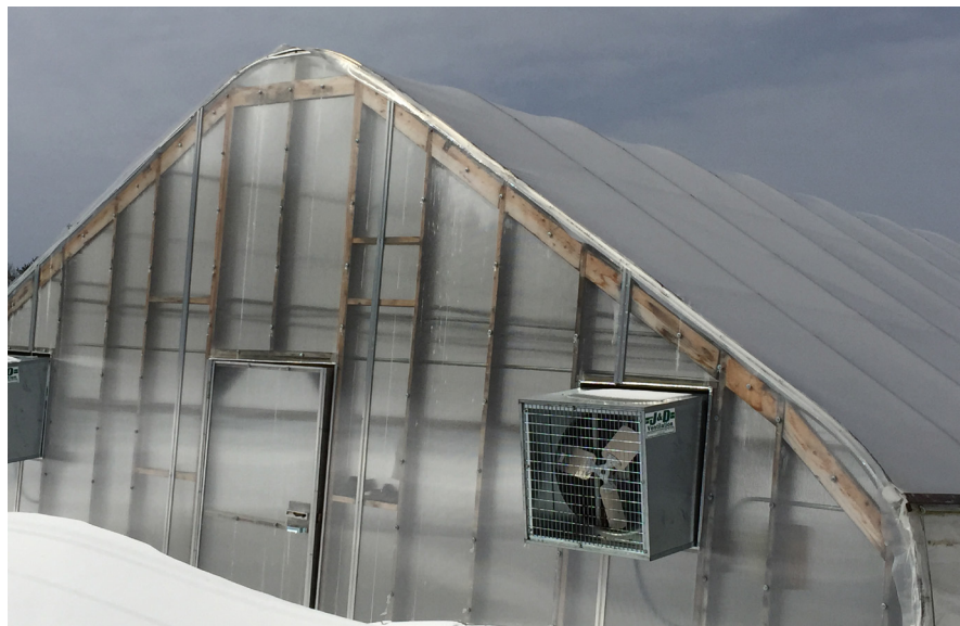
Figure 2. The typical "gothic" design for double-poly greenhouses which does a good job of shedding snow.
