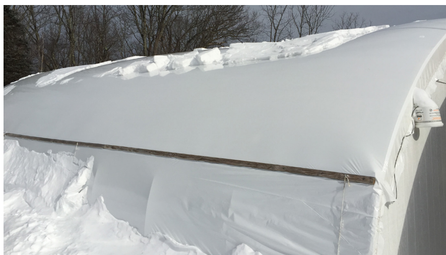
Figure 2. The typical "hoop-house" design for double-poly greenhouses which does not shed snow well.
