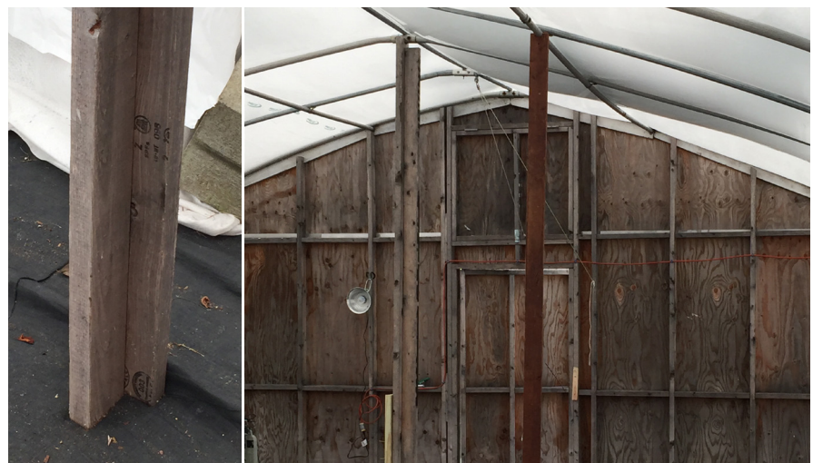
Figure 4. Using 2x4's screwed or nailed together on thier edges to make a "T" can be used a temporary supports for the greenhouse during a snowstorm.
