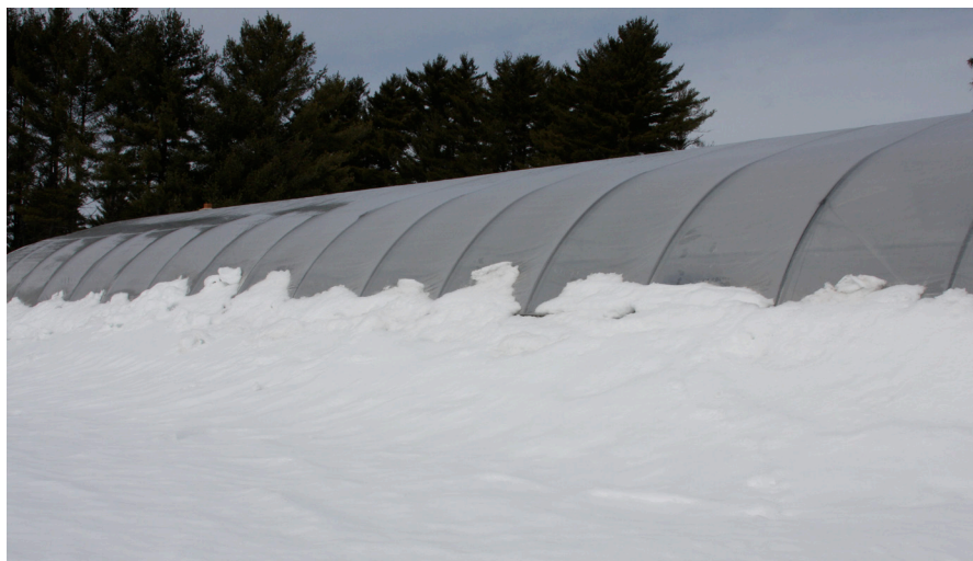
Figure 5. Snow will build up along the sides of the greenhouse and can prevent the snow from being shed from the roof.
